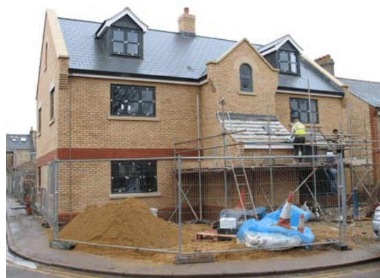
Westfield House - Student Accommodation Center
